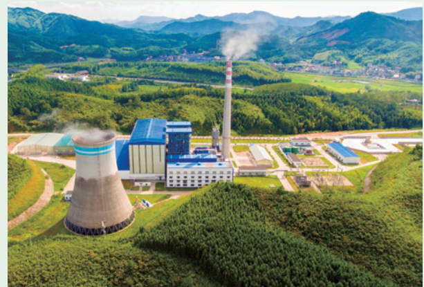
Sunner's New Energy Facility
